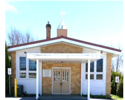
St. John the Baptist Church Port Severn
