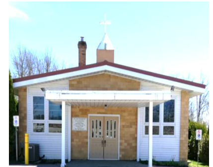
St. John the Baptist Church Port Severn
